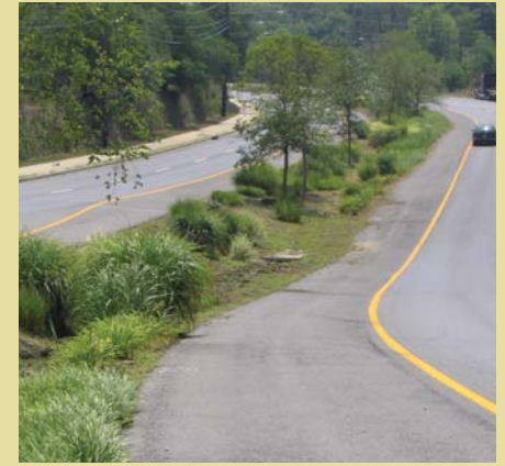
Low impact development median absorbs stormwater runoff from Adelphi Road in Prince George's County, Maryland.
