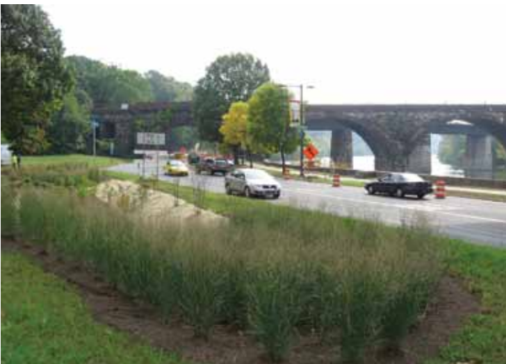
Vegetated bioswales along busy roadsides can capture polluted runoff from impervious surfaces. Source: US EPA
