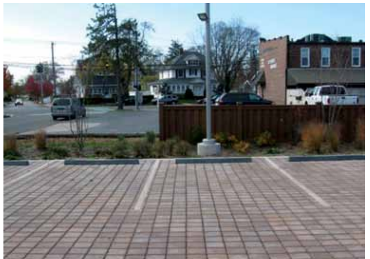
Permeable pavers are a river-friendly substitute to concrete and asphalt. Removing curbs and directing flow into rain gardens captures stormwater. Source: US EPA
